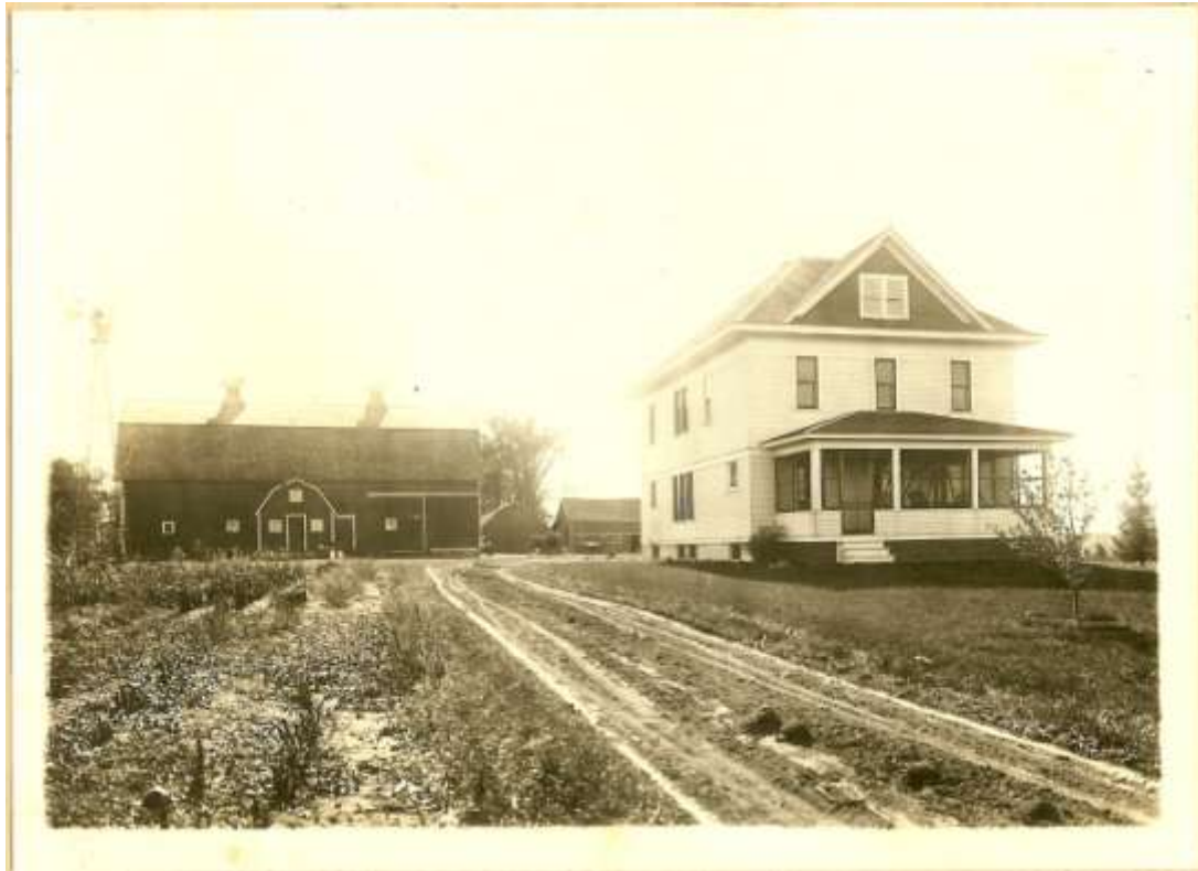
Figure 9-1. Front View of the Kadlec Farm.
