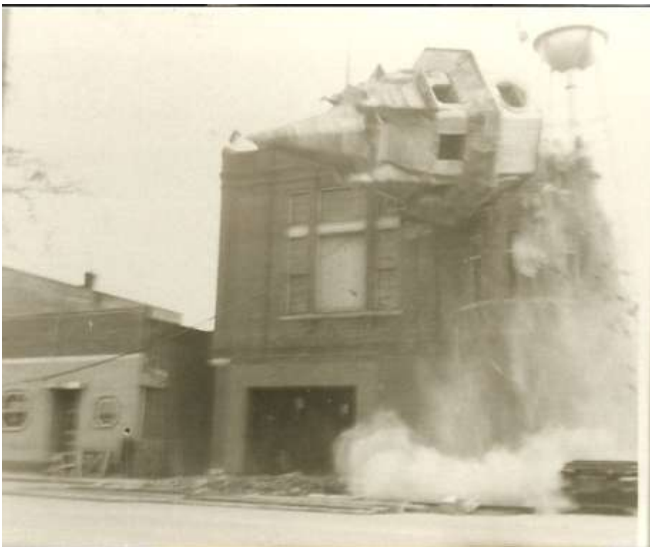
Figure 6-28. Silver Lake Village Hall and Opera House, Razed in 1960.
