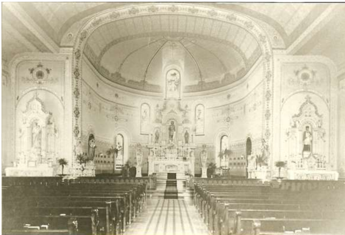
Figure 6-5. St. Joseph Catholic Church, Before 1960's Renovation, Silver Lake, MN.
