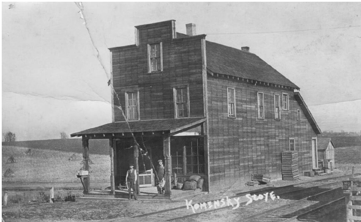
Photo of the Old Komensky Store, looking to the east from the intersection of the Luce Line Railroad and Major Avenue.
